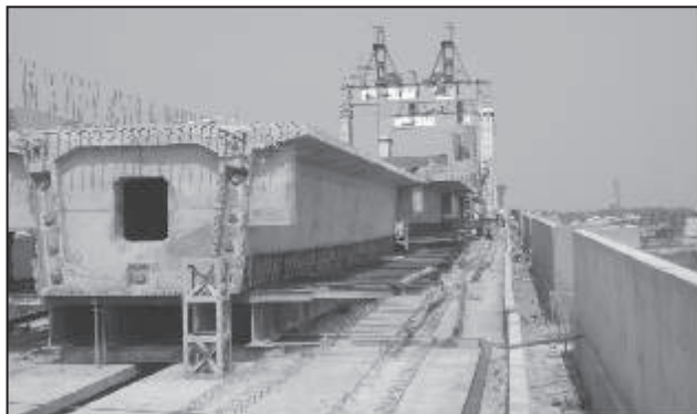
Casting yard with Goliath Cranes on the background
