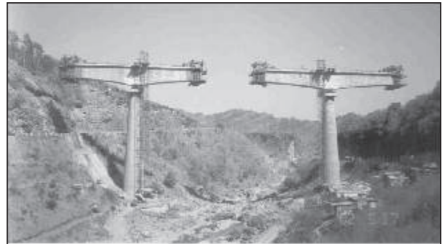
Fig. 17: Balanced Cantilever Construction
