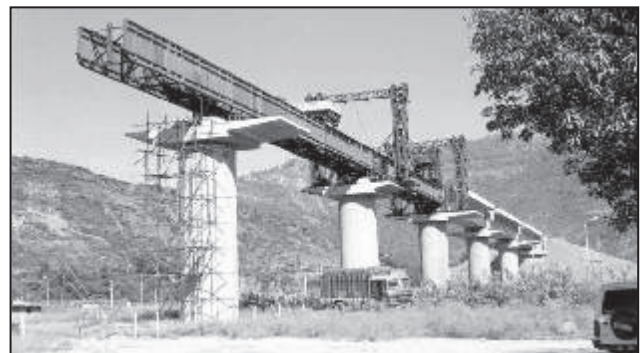
Fig. 18: Launching of 30m Span Precast PSC Box Girder
